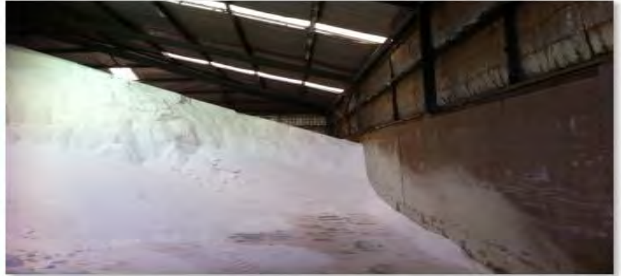
*Sheets corroded through - major falling hazard
