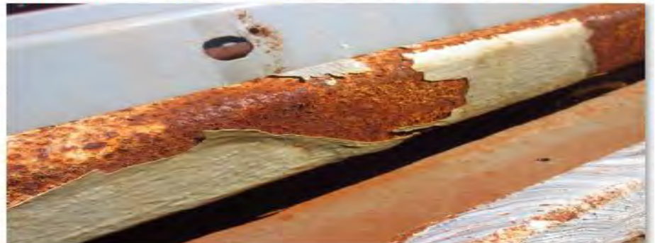
*Tech screws provided entry points for corrosion
