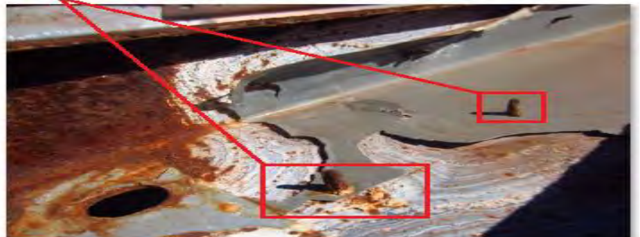
*Tech screws provided entry points for corrosion
