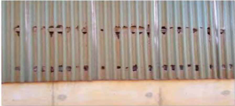
*Roof sheathing corroded in corrugation 'troughs'
