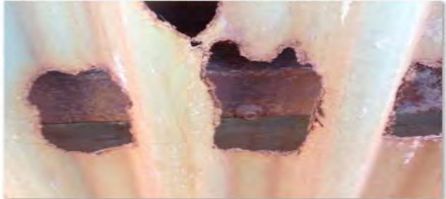
*Internal wall sheathing - imminent risk of falling
