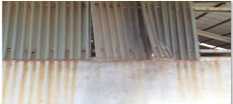
*Internal wall sheathing - imminent risk of falling
